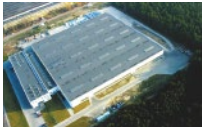
New production plant in Stalowa Wola together with warehouse and the company's new office
